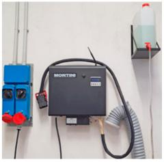
The MONTINI intelligent battery charger automatically adjusts its current to suit the battery capacity, and memorises the need to top up the electrolyte if necessary.
